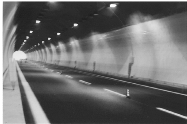
Fig. 3. Casacca tunnel after the rehabilitation of its lining.
